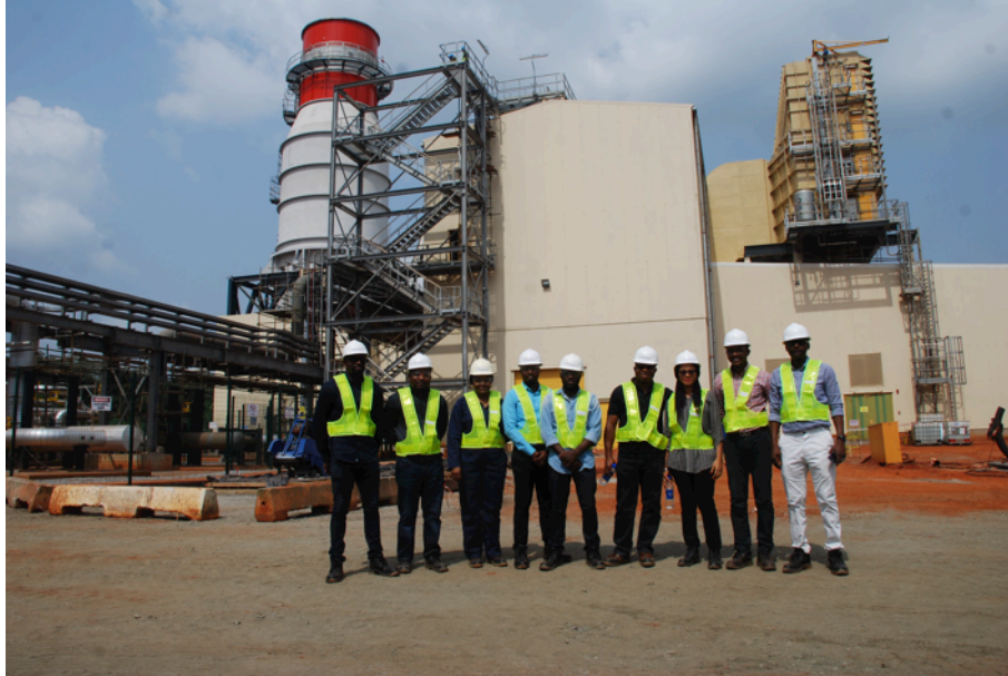
Proud Partners: Staff & management of both Azura and NBET pose by the side of the turbine hall.
